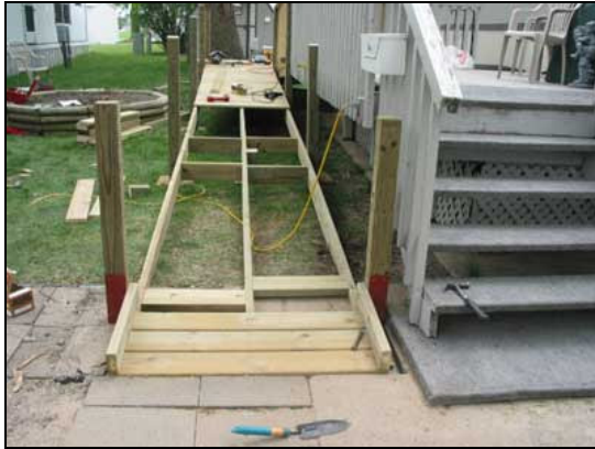
Figure 12. Ramp frame. Notice cross braces.
