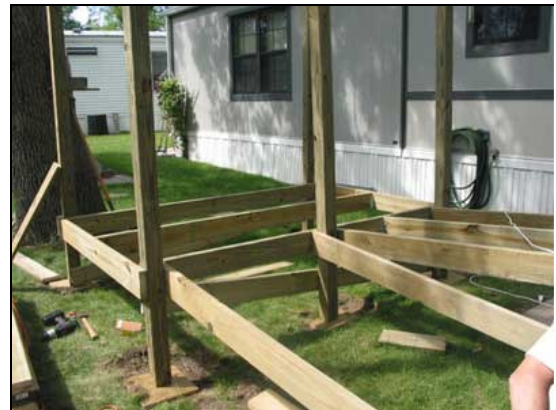
Figure 9. Ramp frame with 180° landing. Notice cross bracing
